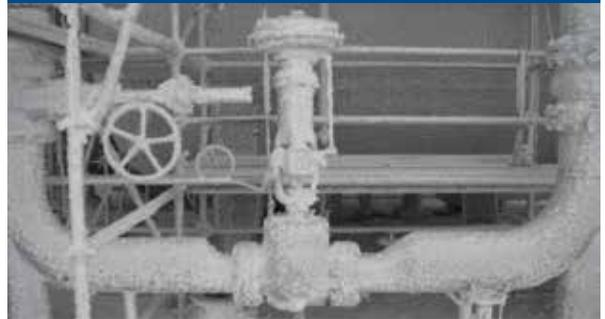
*This control valve photo was taken in January when the temperature was minus 21 Celsius. It illustrates why remote, online monitoring and diagnostics is important to operators at a petrochemical plant in Canada. With a 667 actuator and a FIELDVUE DVC6200-AD instrument, the Fisher ET recycle valve assembly provides reliable flow control for water lines near the cooling towers.*
