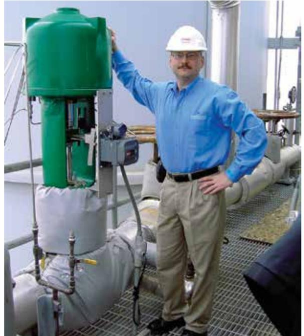
*Fisher® HPT valves with Cavitrol™ III trim reduce cavitation and improve control in boiler feedwater application.*
