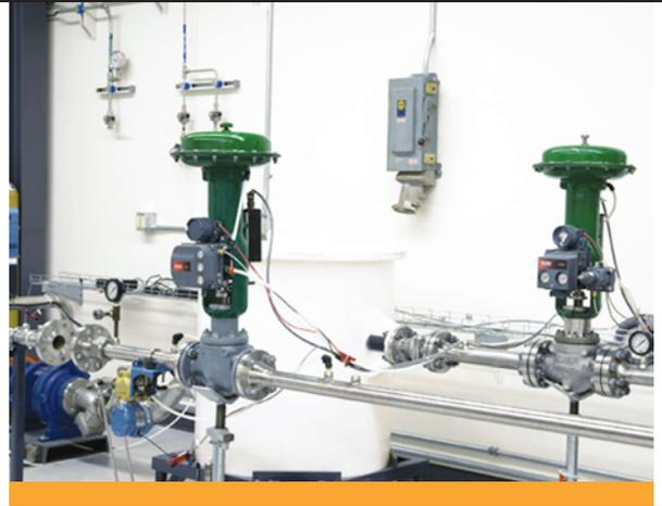
Team Fisher engineered a two-valve solution (like the one used in a differentiation lab (above) to meet severe-service requirements in a silane unit. Two eight-inch, Design ED valves with Inconel body-trim, full bellows, and FIELDVUE DVC6000-PD tier instruments serve a plant producing silicon wafers.
