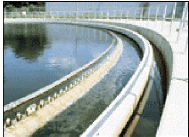
Sedimentation and clarification processes are designed to settle suspended solids in rectangular, circular or conical shaped basins. Tube settlers and plates are used in some shallow basins to reduce the flow velocity and promote settling of the suspended solids.
