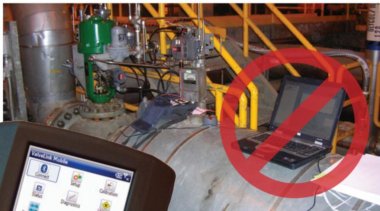
**What a nightmare! Running valve diagnostics in a typical plant used to mean a laptop and tools on top of pipe. Short cables and less-than-ideal valve locations could make the task long, difficult and, sometimes, less than thorough.**
