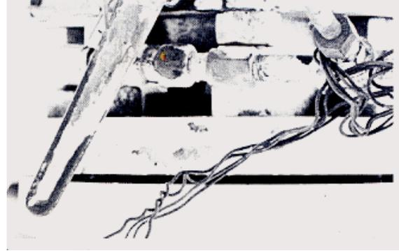
**Figure 5.** Wires like this indicate a lack of valve maintenance. They are used to hold the operating lever open—a very bad practice.
