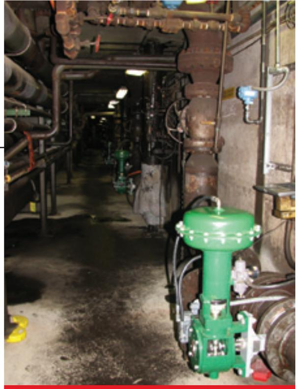
*Up to nine Control-Disk valves, like the one in the foreground, will be installed along this hallway, controlling the flow of water to pumps and spray nozzles.*
