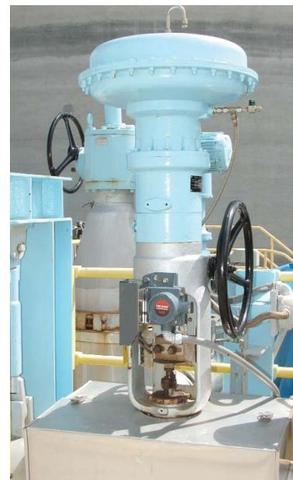
*Feedwater bypass valve with remote mounted feedback sensor*
