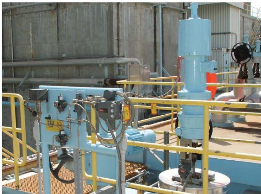
*Feedwater regulation valve with panel mounted instrumentation*
