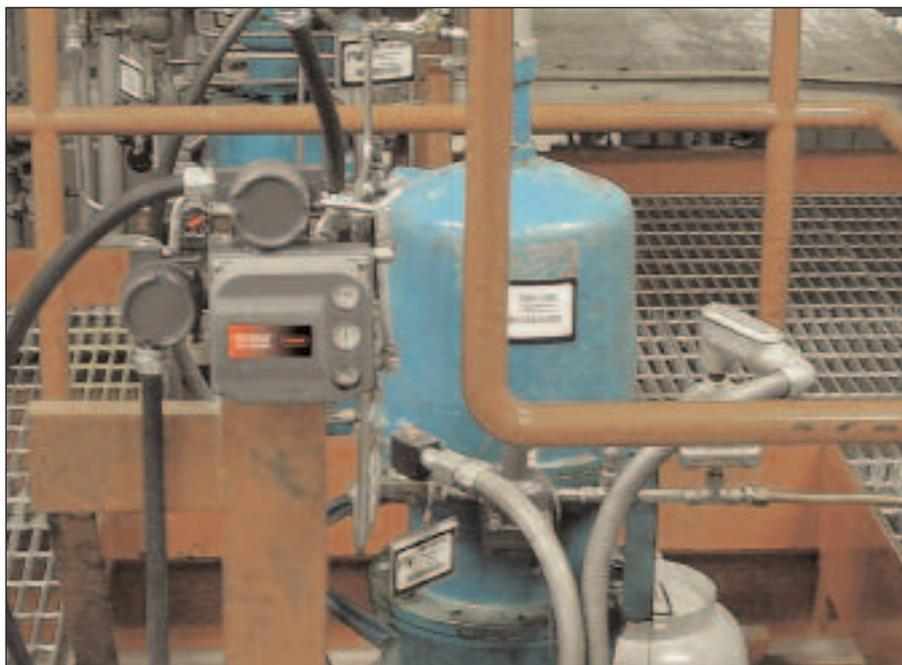
Figure 5. New installation with remote-mounted digital positioner
