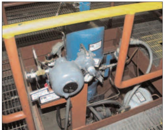
**Figure 3. Original installation, I/P transducer and actuator**
