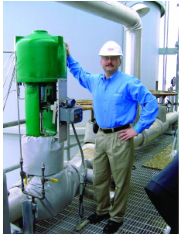
The valve assembly included a FIELDVUE® DVC6020 instrument with Advanced Diagnostics capabilities. The instrument monitors the performance of this critical valve and provides data for its predictive maintenance.
