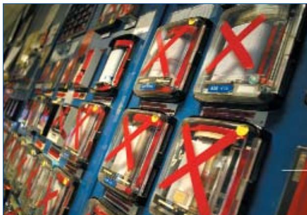
Figure 5. Red tape over old control panel gauges reminds operators as each loop is shifted onto the new quad console.
