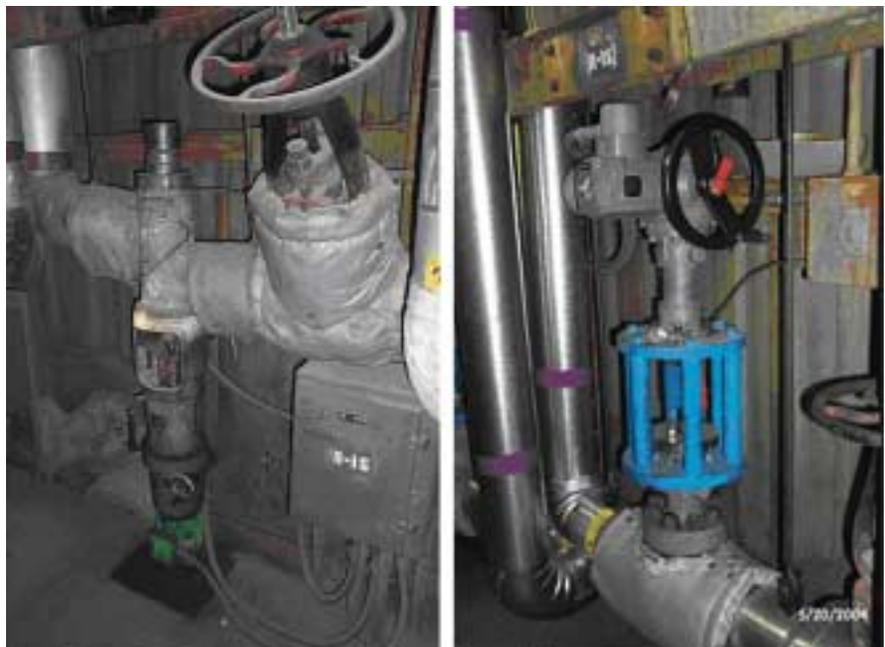
Made at the Fisher service center in Burlington, New Jersey, the valves were installed during an outage in April 2004. They are still working well, without any maintenance problems. The Fisher® EH superheat spray valves provide control within 10 degrees of set point and operate around 60-65% open.
