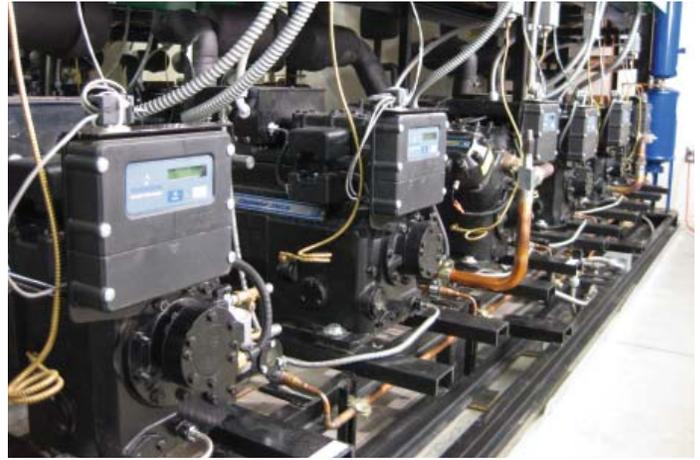
*By integrating several traditional components into one control module, the Copeland Discus Digital compressor with CoreSense Diagnostics modules requires less wiring and fewer connection points, improving system quality and ensuring installation ease and consistency.*
