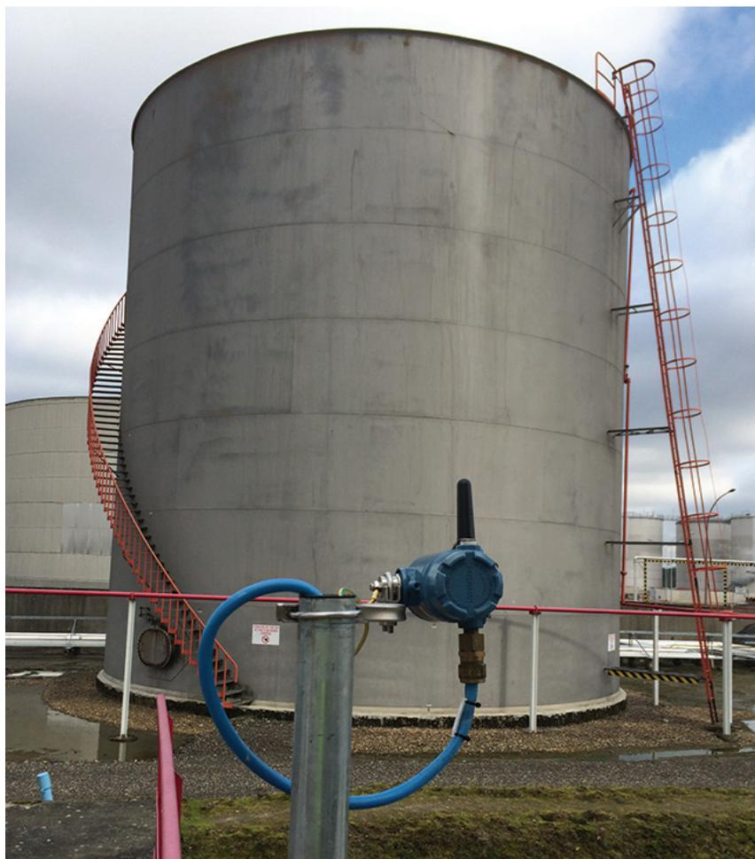
monitoring of critical pumps at the Olefins plant in Teesside," said David Hambling, instrument electrical technical engineer at SABIC UK Petrochemicals. "By installing wireless vibration transmitters we can now continuously monitor vibration levels and detect faults before a failure occurs."
