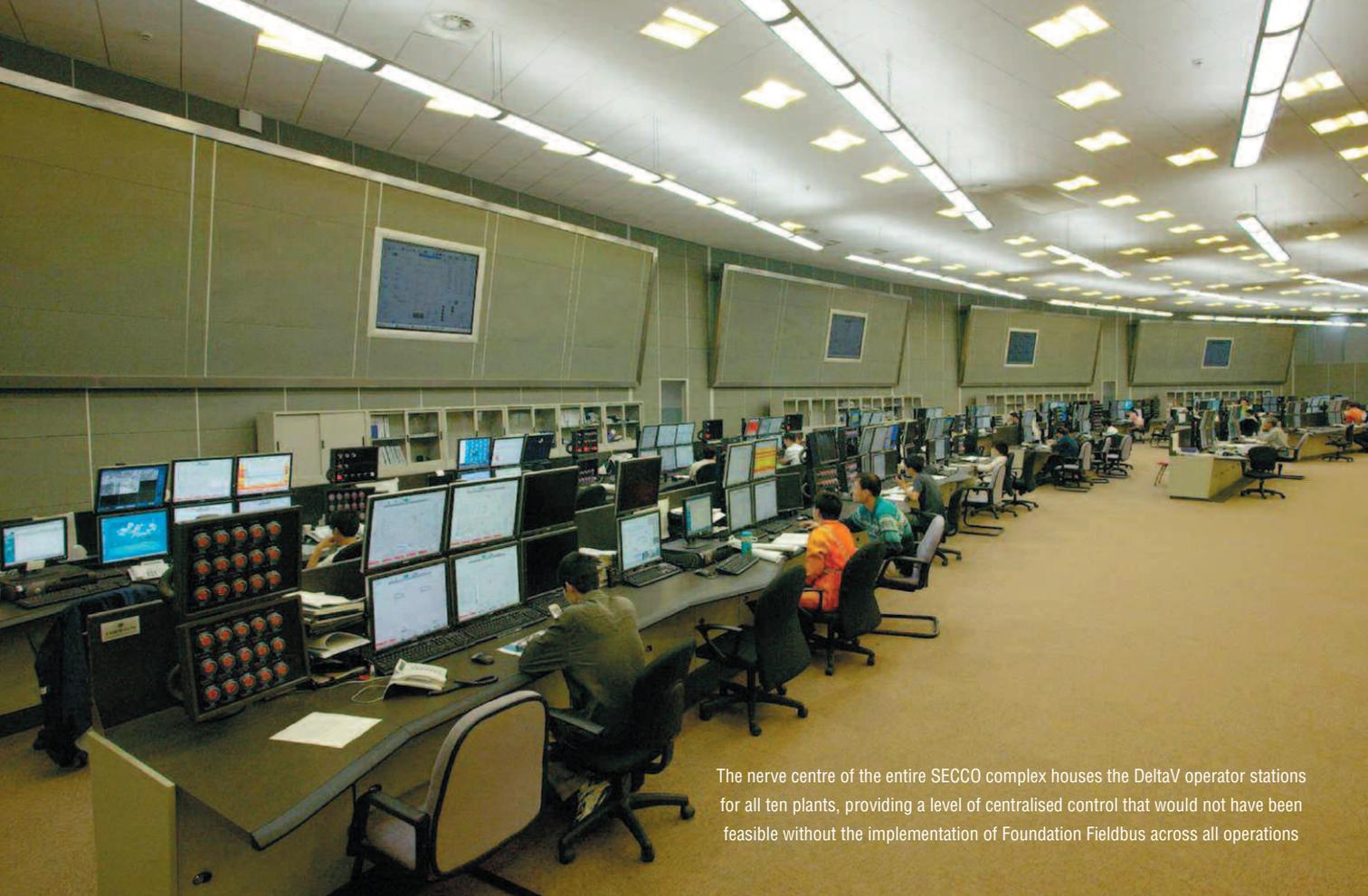
The nerve centre of the entire SECCO complex houses the DeltaV operator stations for all ten plants, providing a level of centralised control that would not have been feasible without the implementation of Foundation Fieldbus across all operations
