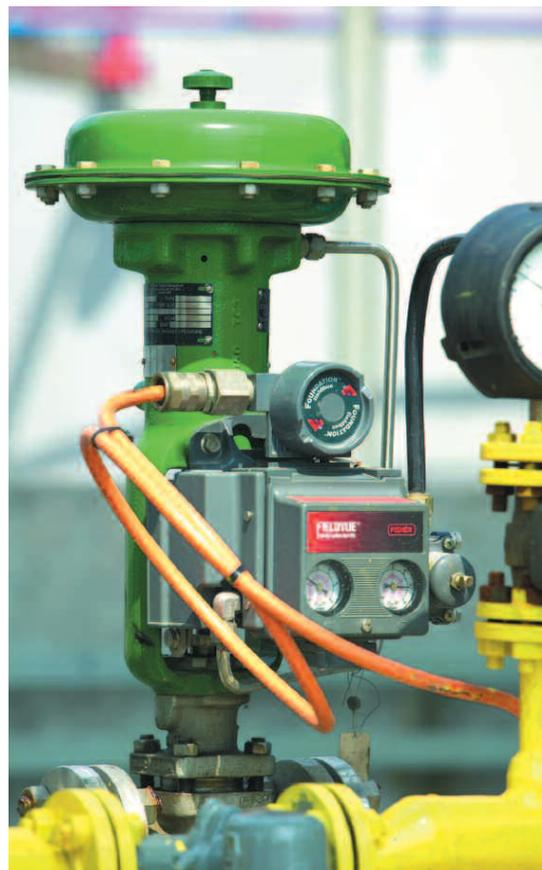
Robust Foundation Fieldbus cabling networks the digital Fisher control valves that feature 'Control in the Field' capabilities with integral PID control
