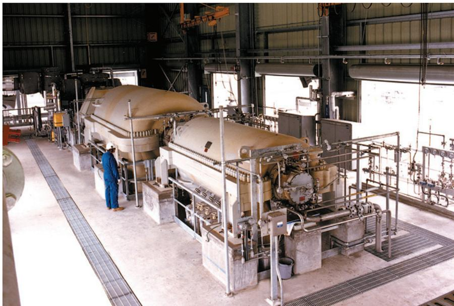
**FIG. 1** The cracked-gas compressor is an ethylene plant's most critical asset. (Photo courtesy of Elliott Co.)
