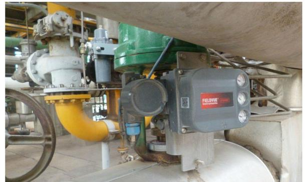
*On the back side of the valve is a FIELDVUE DVC6200 digital valve controller with online monitoring and Advanced Diagnostic capabilities.*
