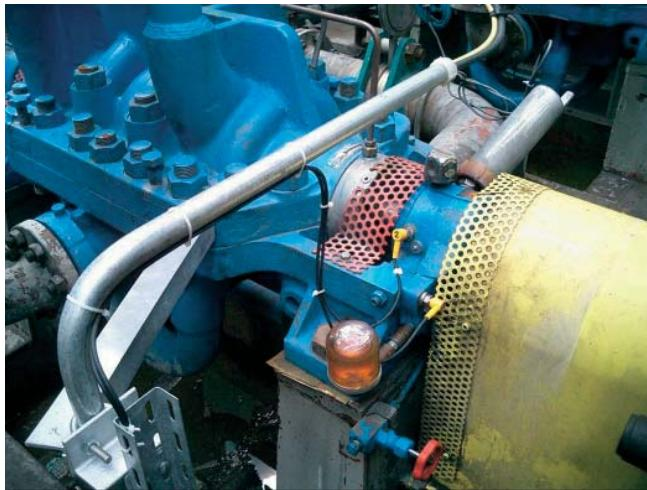
**Sensors monitor changing vibration patterns and rising temperatures in critical pumping systems.**
