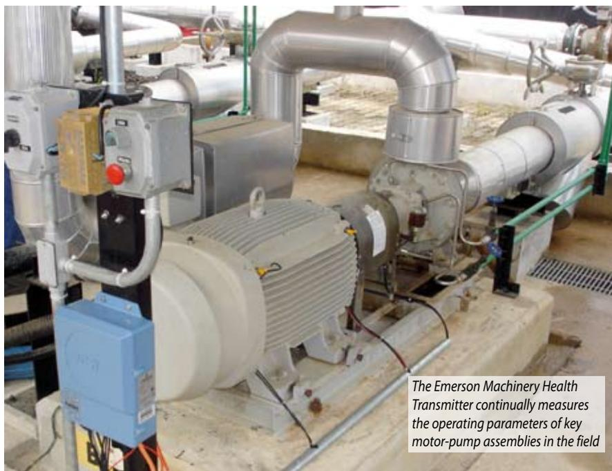
*The Emerson Machinery Health Transmitter continually measures the operating parameters of key motor-pump assemblies in the field*
