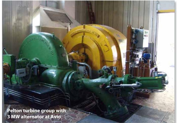
Pelton turbine group with 3 MW alternator at Avio
