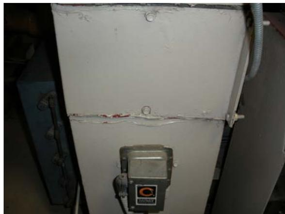
Welded seams from a previous failure serve as a reminder of the value of online monitoring.
