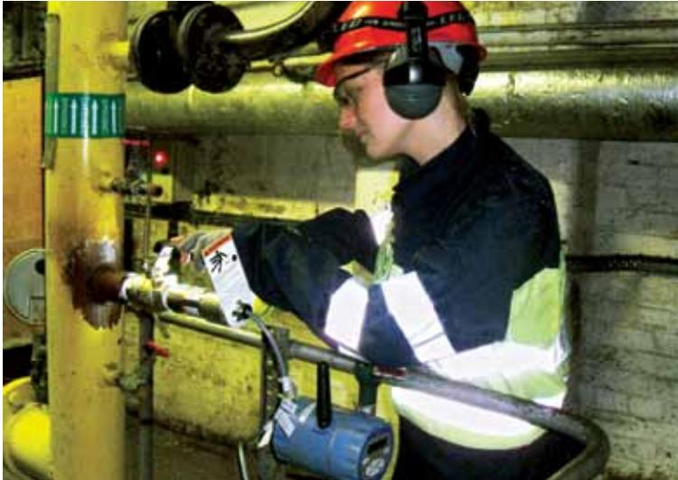
With finite resources, there is often not enough time to manually inspect, clean, and service all the process equipment around the plant to help prevent failures and downtime. The existing primary layer of wired process control for automation, found on the P&ID, is no longer sufficient. Deploying a “second layer” of wireless coverage of missing measurements to automate process equipment inspection, that goes “beyond the P&ID”, can help the maintenance department become more effective.
