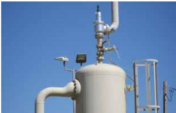
Figure 1: An acoustic transmitter turns an ordinary relief valve into a smart relief valve.
