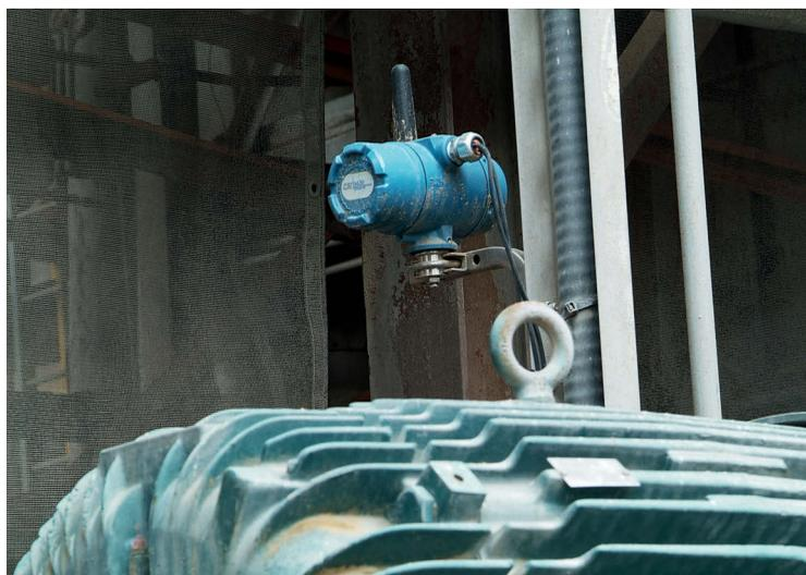
**By installing wireless transmitter to a typical pump this will provide an operator with the multi-parametric information needed to build a clear picture of its health and also that of the process**
