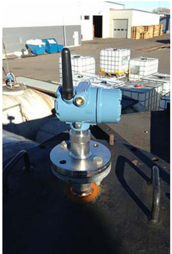
*Figure 2. A battery-powered wireless instrument requires no signal or power wiring, and can operate for up to ten years before the battery needs replacement.*
