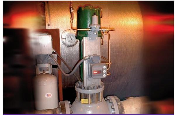
***"We now have FIELDVUE DVCs on the toughest applications in this plant, including the valves controlling desuperheating spraywater, boiler feedwater, dearator inlets, and the soot blowers. They helped identify soot blower valve leaks that were losing as much as \$250,000 worth of steam per year. These losses were eliminated through a combination of corrective actions."***
