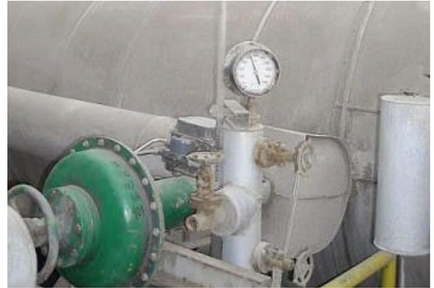
*Wireless transmissions enable continuous monitoring of the performance of key control valves.*
