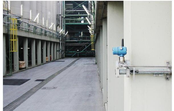
*Eight Rosemount 3051S DP wireless transmitters were installed at the INEOS plant in Cologne.*
