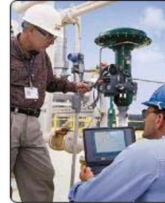
PC tools can speed valve diagnostics in the field.
