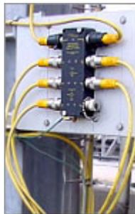
These junction boxes come with connectors for four to eight devices, plus connectors for segment-in and segment-out. Each connector is labeled to help prevent incorrect assembly. Caps protect unused connectors from the environment.
