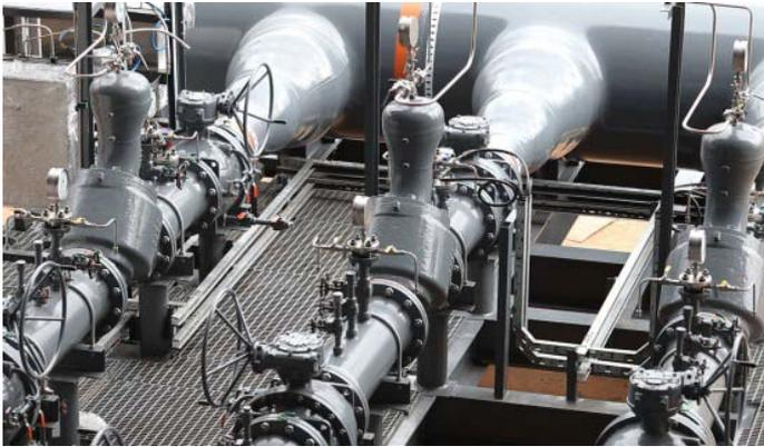
Figure 6: Complete surge relief systems can be provided on a skid, minimizing on-site construction.
