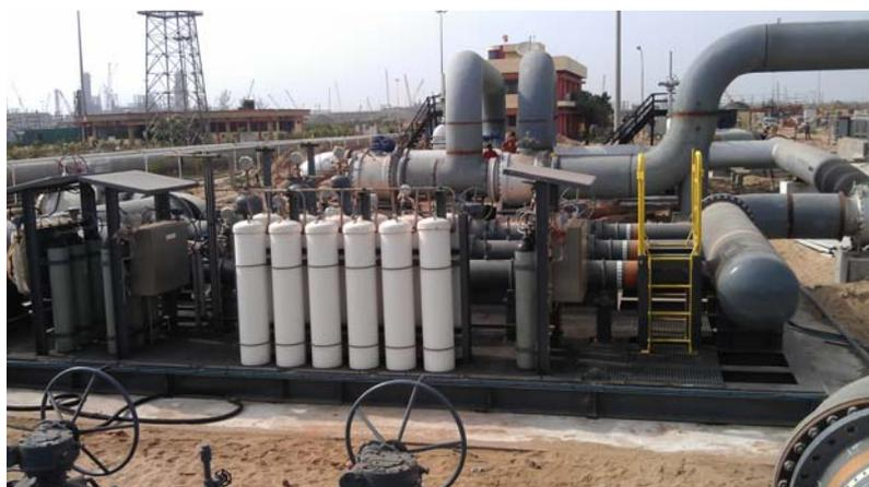
Figure 2: A surge pressure relief valve is an integral part of a complete surge relief system in a pipeline.
