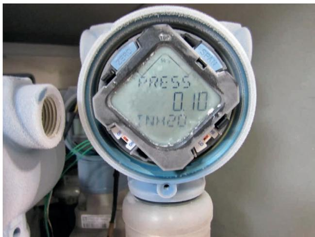
Figure 2. Instrumentation suppliers have improved the electronics used in transmitters, expanding the range of temperatures in which they can operate without problems; courtesy of Emerson Process Management.
