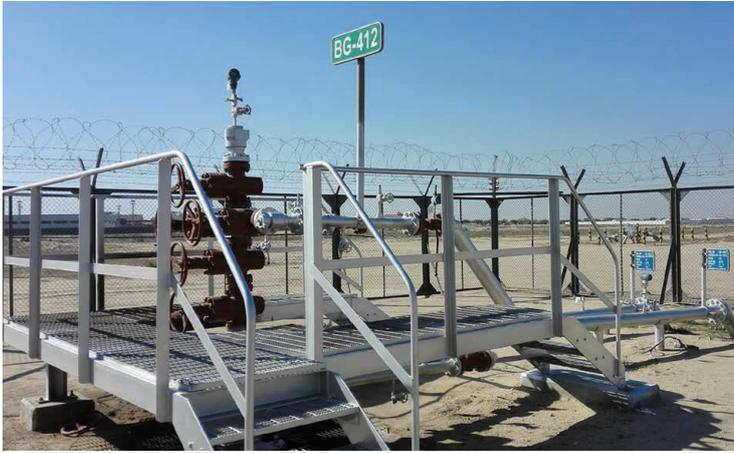
**Figure 1.** This lift station is similar to many others used by KOC. A wireless transmitter measures wellhead pressure, and a second wireless transmitter measures wellhead temperature. Readings from these and other devices are transmitted to and shown in the main control room.
