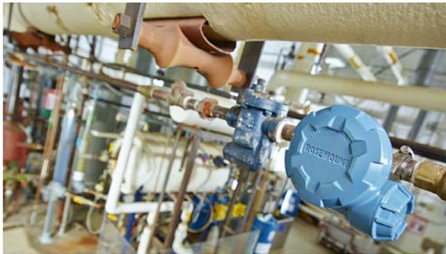
Wireless transmitters measure the ultrasonic acoustic behavior and temperature of steam traps, and send this information to maintenance personnel via a wireless mesh network ensuring high reliability of transmitted data. Because no wiring is required to the transmitters, they can be installed for a fraction of the cost of a wired instrument.
