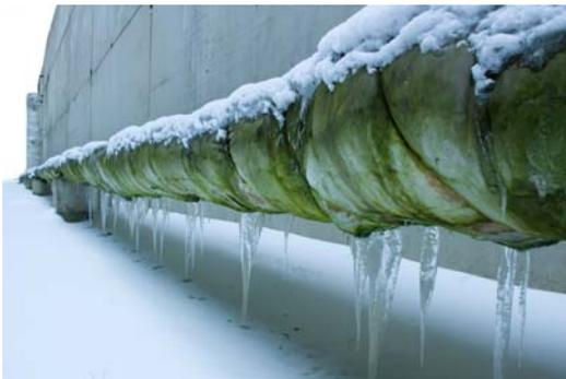
Properly-functioning steam traps are essential for good performance of a steam system. Trap failures compound one another and lead to a range of potentially-serious operational issues. One such issue, common in processing facilities, is freezing of equipment during periods of cold weather. The following are some examples:
