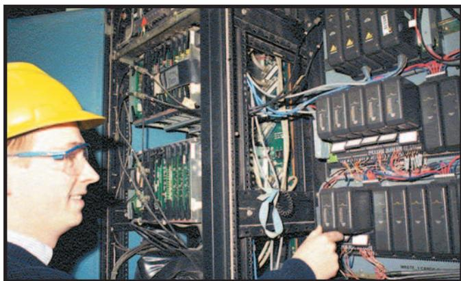
Carl Stumpe checks a DeltaV controller's analog I/O module. The controller is mounted in cabinet space that used to hold DCS equipment.
