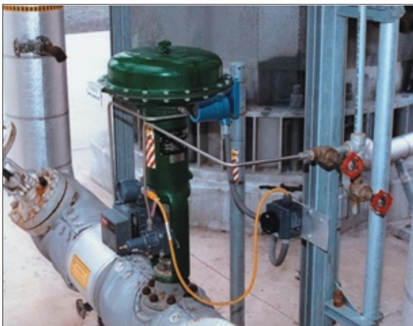
A termination of a fieldbus spur on a digital valve controller takes the PID logic out of the process controller.
