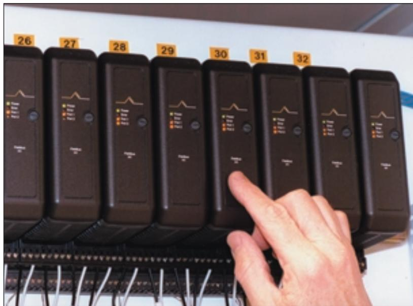
A bank of fieldbus control and I/O modules, shown here, offers fully distributed logic.
