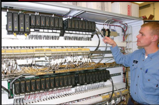
Figure 2. This new cabinet houses a controller and I/O for a portion of the acrylonitrile unit. CPU and power supply modules (upper left) are redundant.
