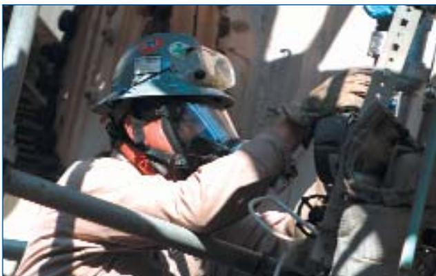
Figure 4. Hot cutovers of transmitters required only the repositioning of process measurement tubing from old to new.
