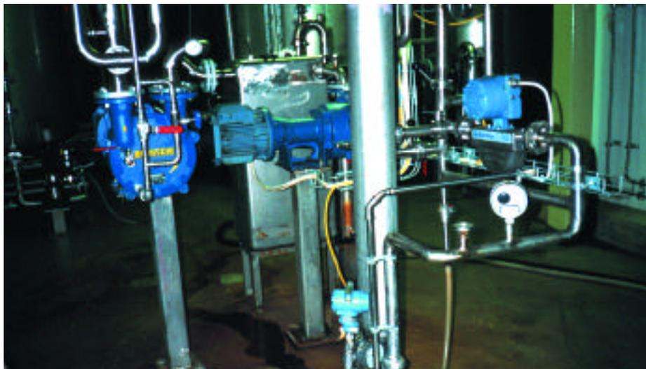
**Coriolis mass flow meters, pressure and temperature transmitters, and pH transmitters communicate with each other through FOUNDATION™ fieldbus and the DeltaV system.**
