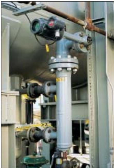
Pneumatic transmitters on displacer level sensors were retrofitted with intelligent transmitters communicating via HART digital traffic superimposed on a conventional 4–20 mA analog signal (Fig 11).
