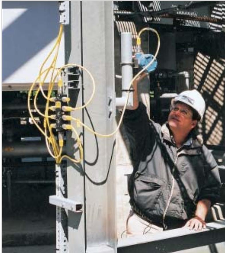
Verret points out a typical intelligent transmitter connected to a Foundation fieldbus segment at the "brick" on the column (Fig 10).
