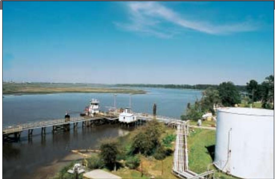
based on electromechanical relays and timers. The tank farm had no remote instrumentation or control, instead using locally indicating float gauges and manually operated pumps, valves, and local pneumatic controllers.
