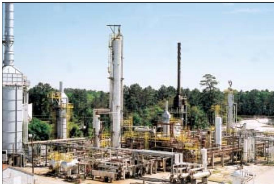
Processing portion of the Calcasieu refinery, Crude Unit No. 1 and naphtha stabilizer (right) and Crude Unit No. 2 (Fig 1).
