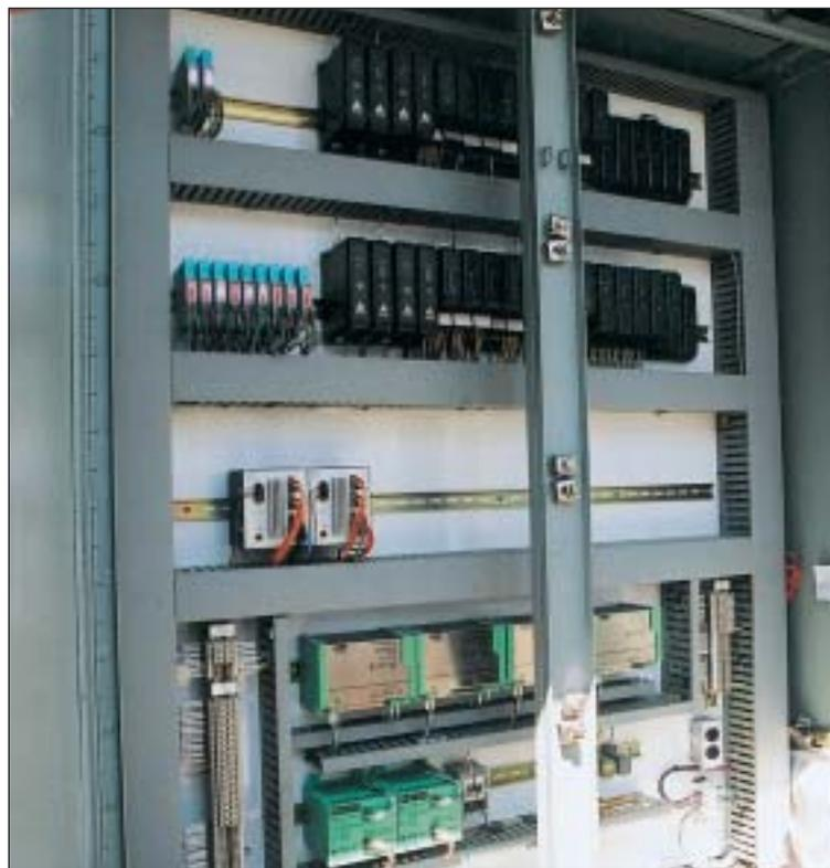
Field-mounted DeltaV controllers and I/O modules for the naphtha stabilizer, top row also serving the tank farm and pipeline, and Crude Unit No. 1, second row (Fig. 8).
