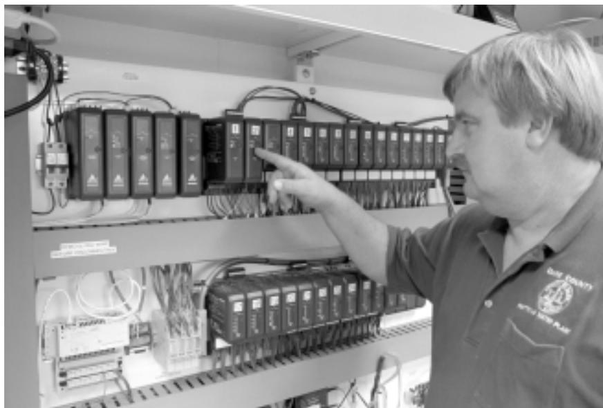
*Flatt checks the operation of the digital process automation controller running the entire water treatment facility. This controller is a key component of the field-based automation architecture.*
