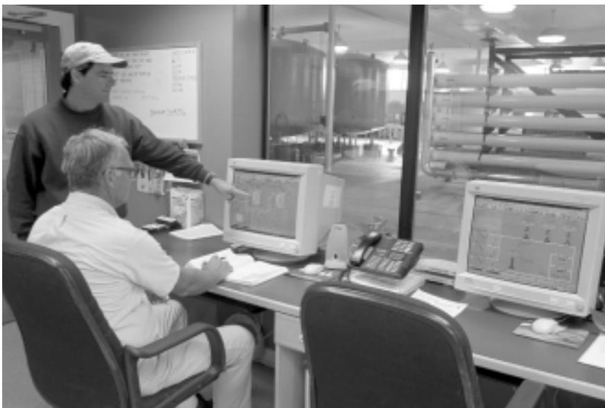
Plant Superintendent John Contestable (standing) and Plant Operator Chuck Ethridge monitor operations at the PC workstation. Through the window they can view the anion exchange vessels (left) and reverse osmosis units.
