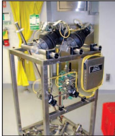
**Cleaning bioreactor units requires a portable valve cart to be hose-connected manually to various process piping headers on the bioreactor.**
