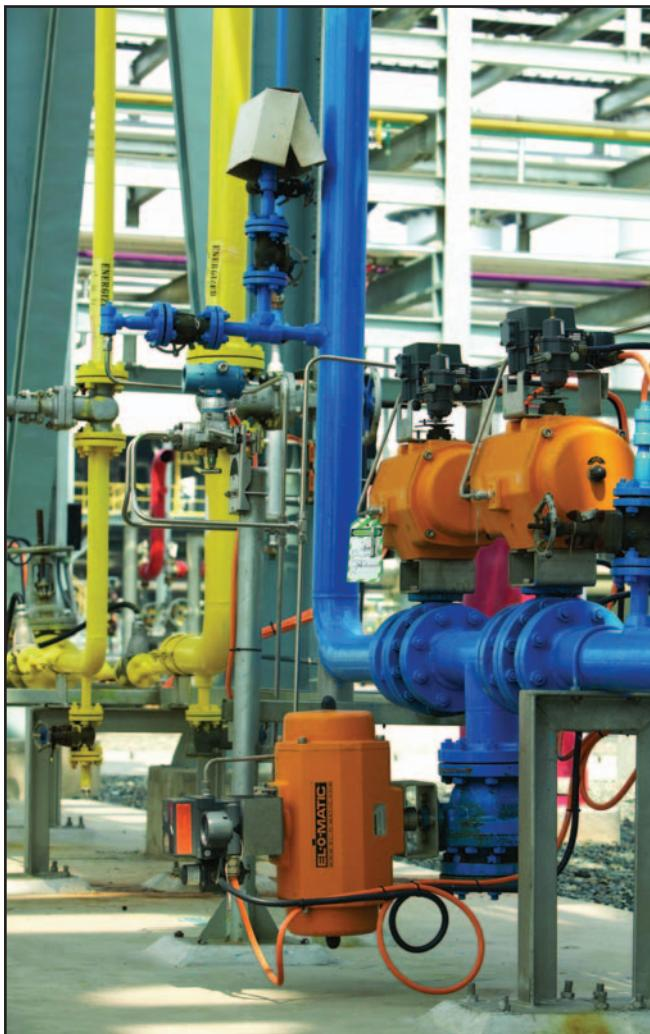
**Fieldbus and smart valves permit locating the controller in the control valve, distributing control to the exact point it is needed.**
