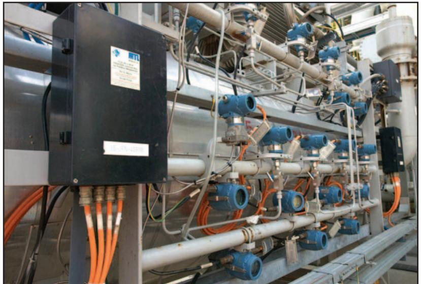
**More than 20 differential pressure transducers connected via Foundation Fieldbus, saving wiring cost and making operation easier.**
