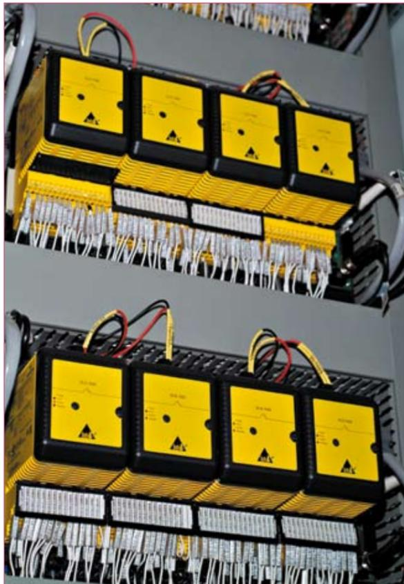
Figure 2. DeltaV SIS logic solvers installed on Rompetrol's distillation fired heaters.
