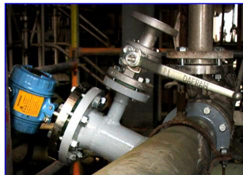
Figure 1. Micro Motion® Direct Insertion Fork Density Meter installed at company location.
