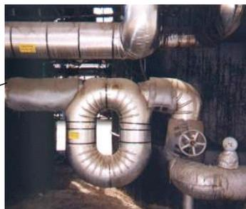
*CMF400 enclosed in an insulated heat jacket*
