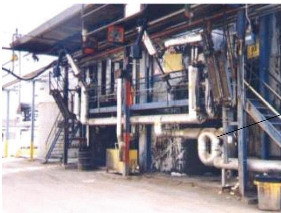
*Asphalt loading with Micro Motion CMF400 meter installed*
