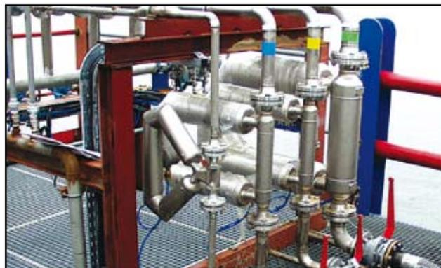
**Figure 6. Micro Motion Elite meters of various sizes in use at LBC Tank Terminals in Antwerp.**
