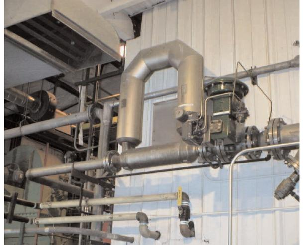
*This Micro Motion Coriolis meter accurately measures gas flow regardless of composition, allowing the plant to switch between different fuel gases.*
