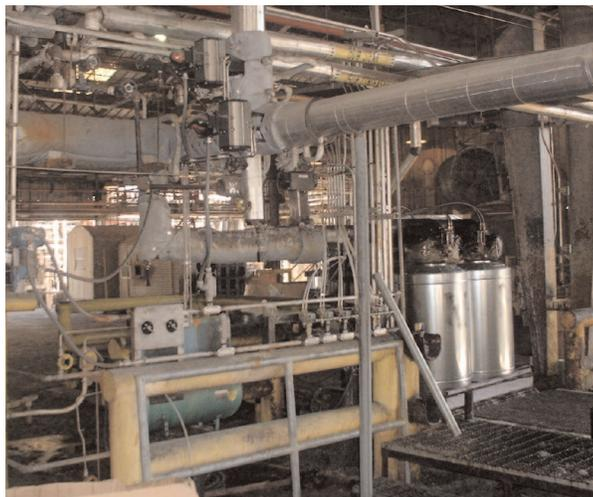
*A Micro Motion meter measures the flow of hot rosin into drums.*
