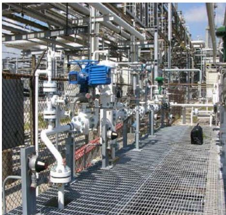
Metering skid with Micro Motion ELITE meter installed for critical phase ethylene custody transfer
